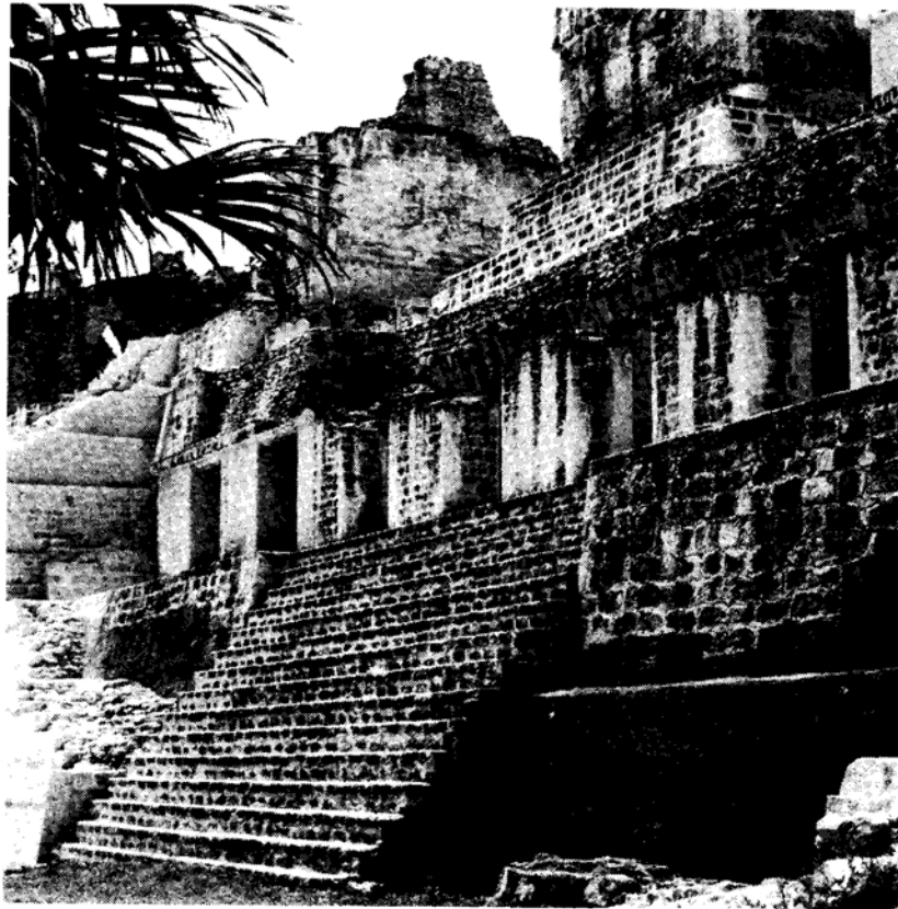
At the South side of Great Plaza: nine door-way building. (Structure 5D-120.)
