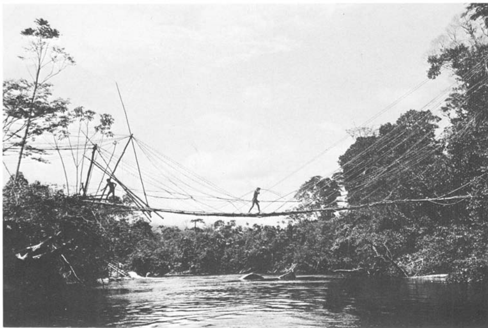
Fig. 3. 40-meter long bridge of jungle vine across the Maturacá river, made by the Yanomamö Indians of the village of Caburiwe-teri.
