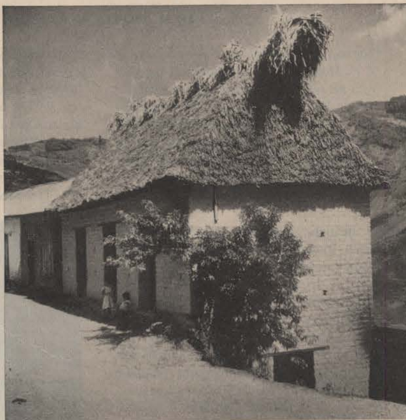
HOUSE where mushroom sessions took place is built of adobe, has thatch "dog-ears" over gable ends. Door, lower right, leads into ceremonial room.
